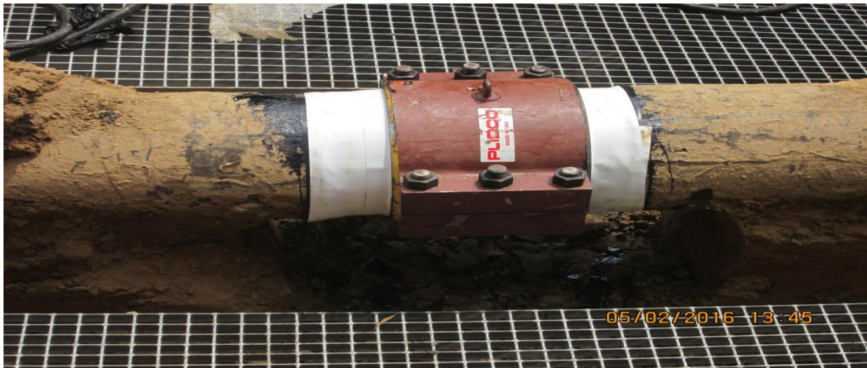
FIG 7: Clamp job completed
